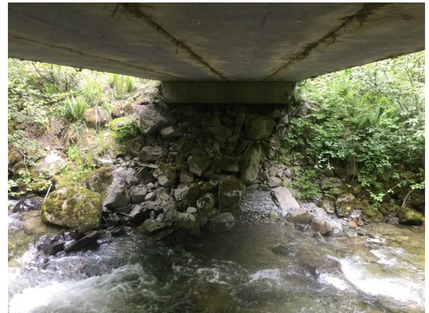
Left Bank Abutment when facing downstream
