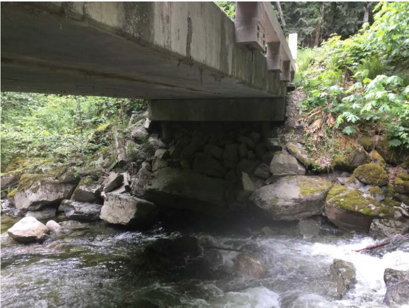
Right Bank Abutment when facing downstream
